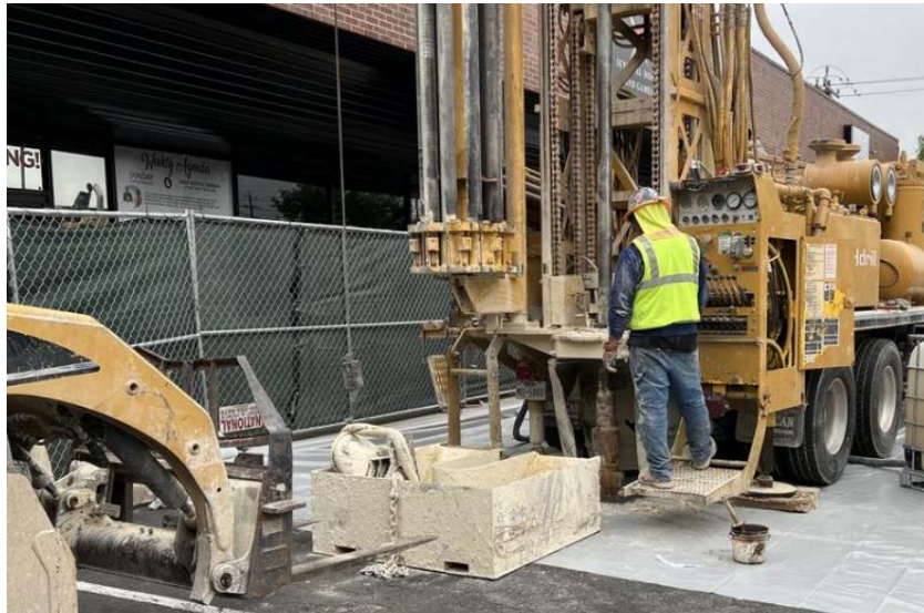
Photograph #2: Installation of a horizontal SVE well in progress.
