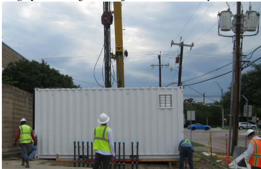
Photograph #3: Lifting and setting one of the treatment system containers.
