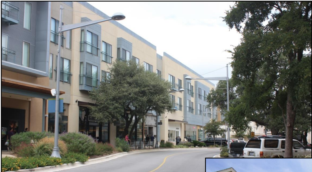
Multi-family above retail in a mixed use development
