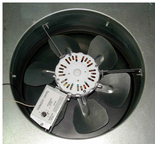
Figure 7 – Control box of 10N201 was mounted on the base.
