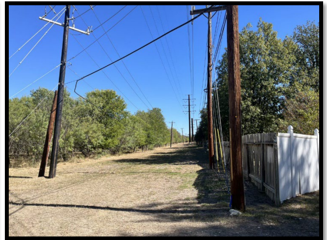
Figure E. Fuels reduction around power lines and residential properties significantly reduces wildfire risk.
